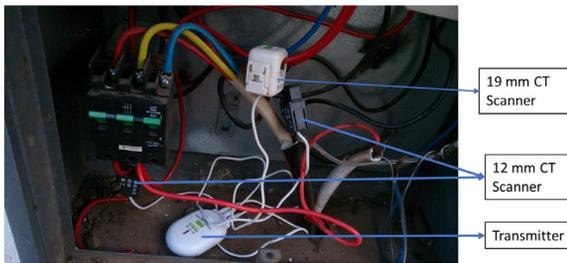
**Fig. 4.** CT scanners and transmitter
