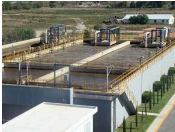
Reactor aerobio
