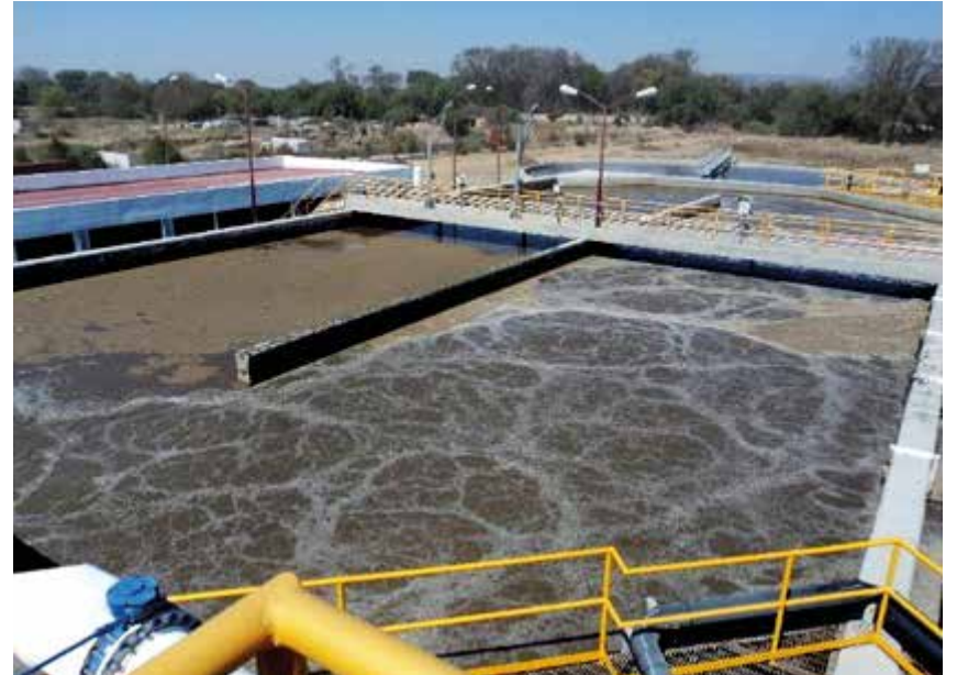
Reactor aerobio
