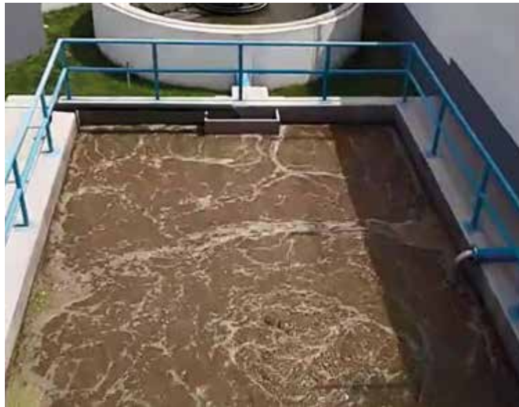
Reactor aerobio
