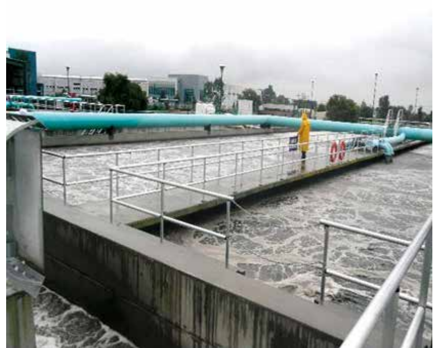
Reactor aerobio
