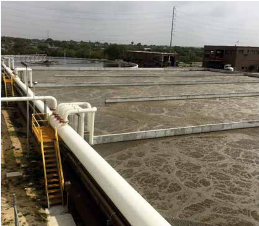
Reactor aerobio
