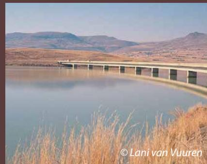
*The Sterkfontein Dam stores water for release to the Vaal River. Water is sourced from the Tugela River and pumped upwards from the Woodhead Dam. The Vaal and Sterkfontein Dams are among the top five largest dams in South Africa at present.*
