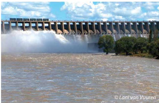
*The Vaal Dam wall was initially 54.2 m at the lowest foundation and is a gravity dam comprising a concrete gravity structure with an earthfill section on the right flank. The height was increased to 60.3 m in the 1950s, and again to 63.4 m in the 1980s. The dam presently stores roughly 2 600 million cubic metres of water with an additional temporary flood safeguard just above 600 million cubic metres.*
